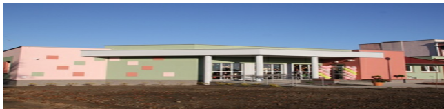
Construction of a kindergarten in Stare Oborzyska
